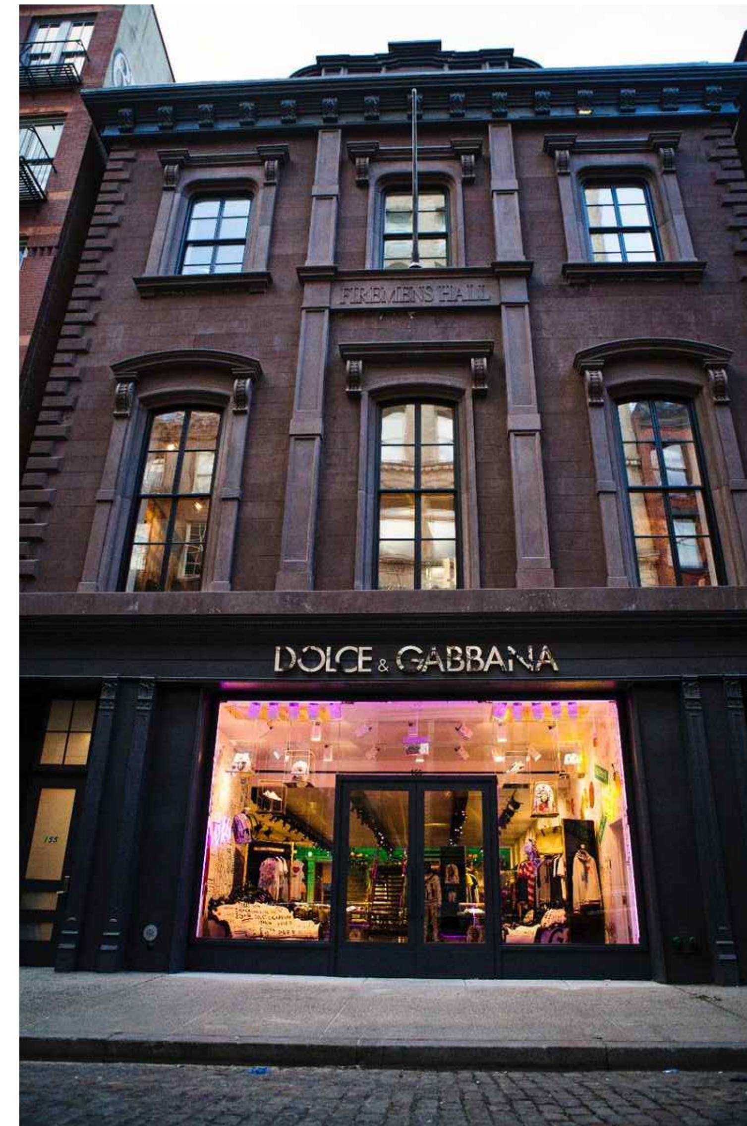
STOREFRONT WITH NEW PURPLE NEON PERIMETER ACCENT LIGHTING INSTALLED ON STOREFRONT GLASS FRAME – VIEW 2
