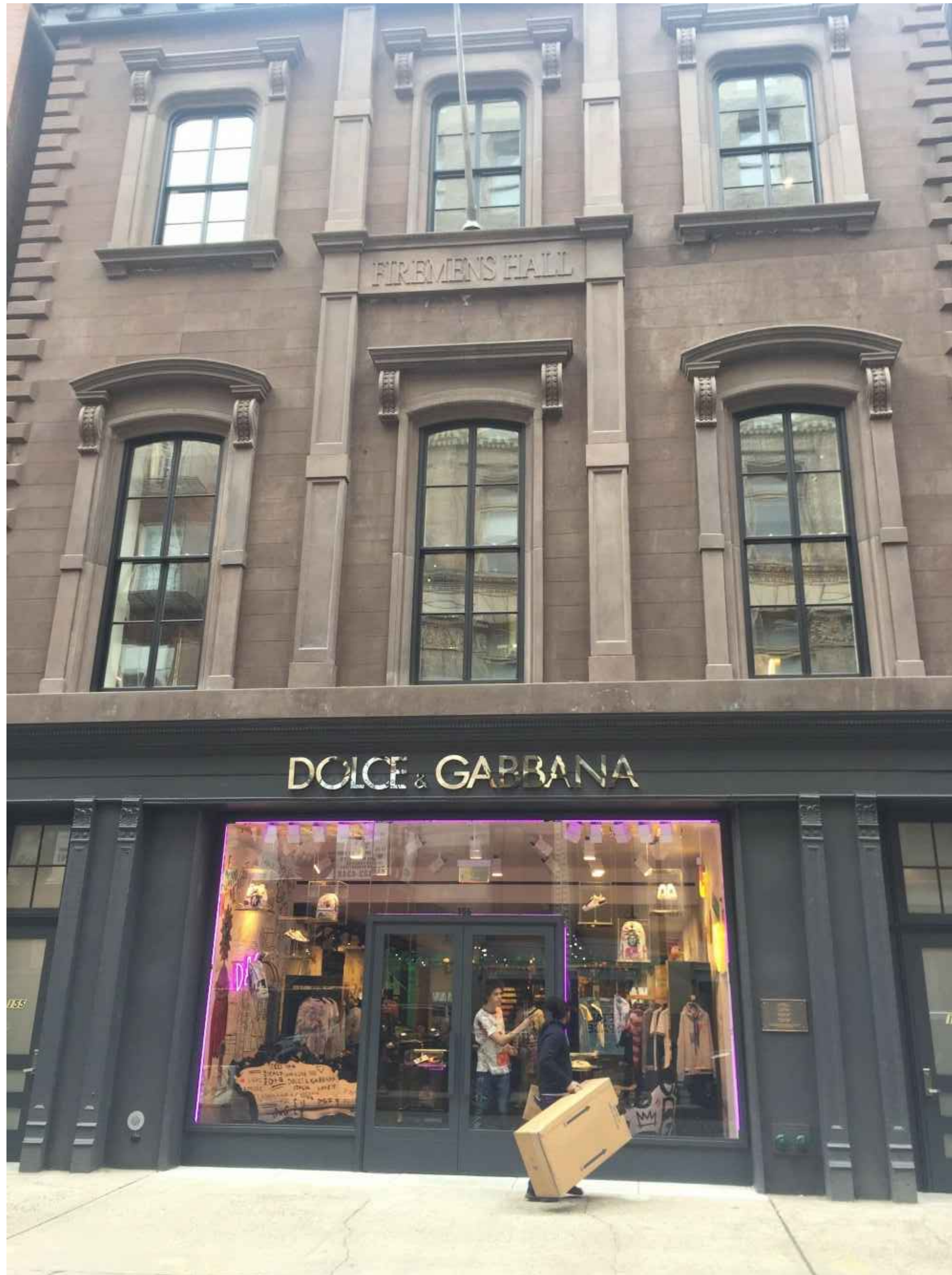
STOREFRONT WITH NEW PURPLE NEON PERIMETER ACCENT LIGHTING INSTALLED ON STOREFRONT GLASS FRAME – VIEW 1
