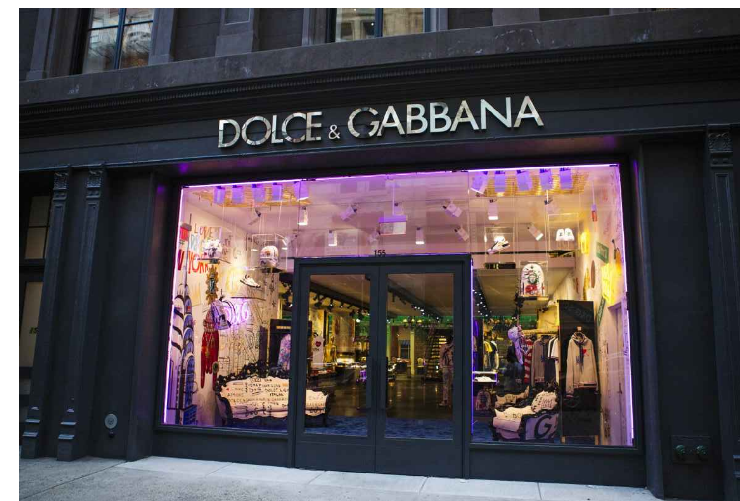
STOREFRONT WITH NEW PURPLE NEON PERIMETER ACCENT LIGHTING INSTALLED ON STOREFRONT GLASS FRAME – VIEW 3
